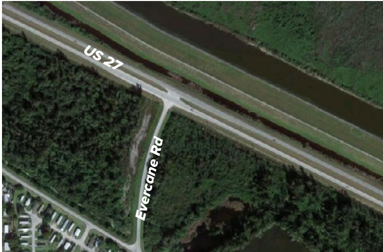
Aerial depicting current intersection configuration
