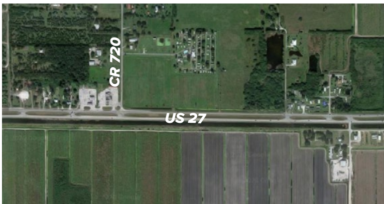
Aerial depicting current intersection configuration
